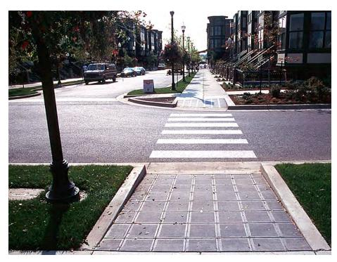
An example of an intersection with separated ramps and landings and clearly defined pedestrian crosswalks.
